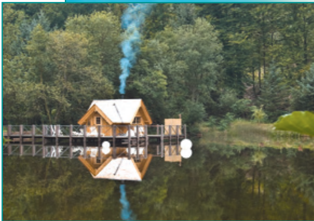
New Sauna on pillars in Swimming Lake
